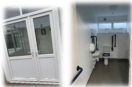
New front/internal doors
